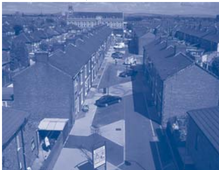
Stainer Street, Northmoor, Manchester. The first home zone in the UK showing a shared surface treatment, indirect vehicular route, parking arranged in echelons, patterned paving and street tree planting.
